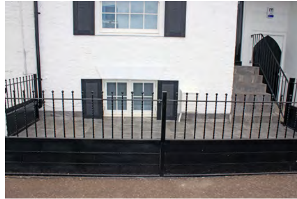
Paved over front garden reducing opportunities for the addition of greenery
