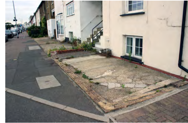
Front gardens converted to parking with the loss of boundary treatment
