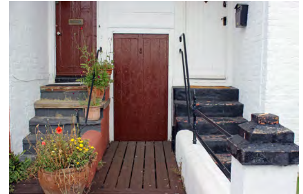
Parts of original railings remaining at No.44 (left) and No.45 (right)
