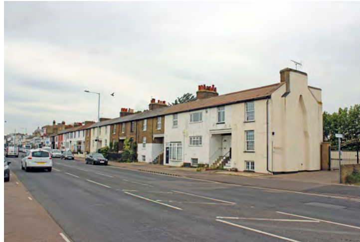
View looking north-west
